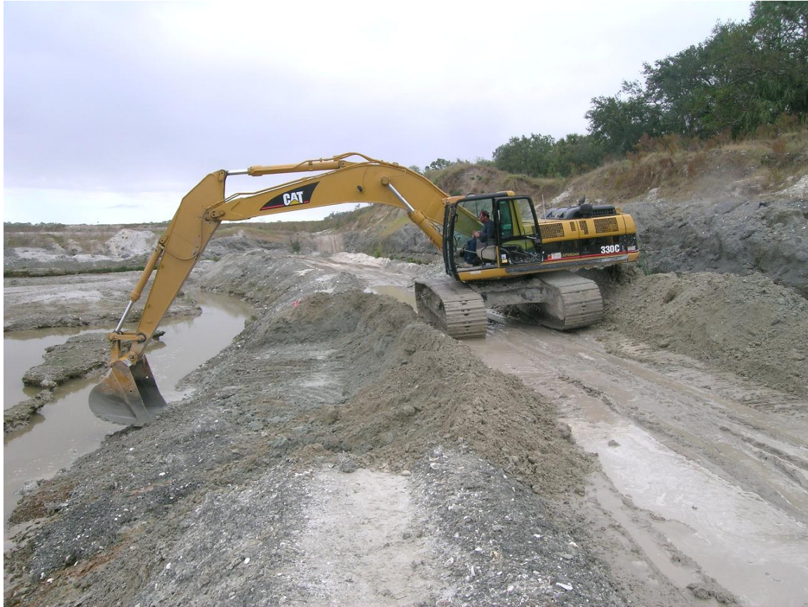
Figure 6: Track hoe removing overburden from above the basal Mercenaria permagna zone
